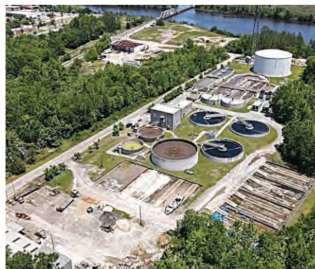
Photo courtesy of the City of Milton. Milton's current wastewater treatment plant.
